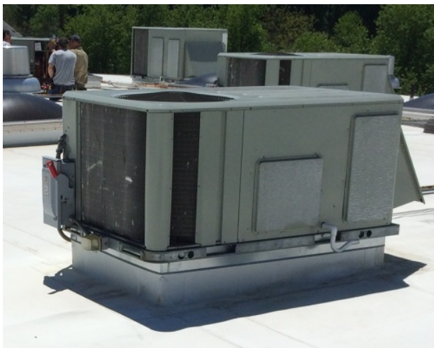
Figure 15. Roof-top HVAC unit
