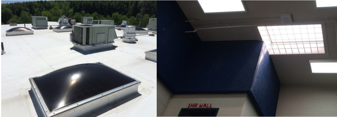
Figure 14. Skylights on the WCDF
