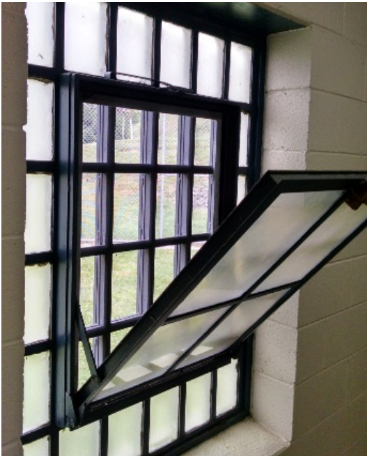
Figure 11. Window in Building B.
